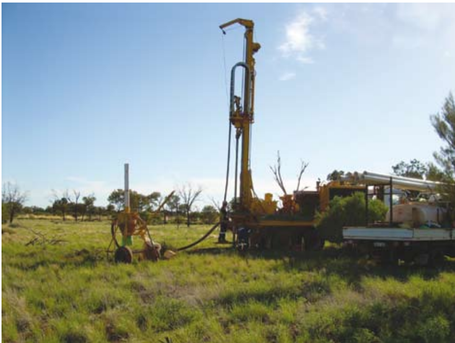
Air core drilling at McPherson’s Bore.
